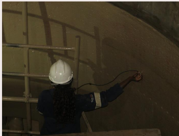
Paint thickness testing - draft tube
