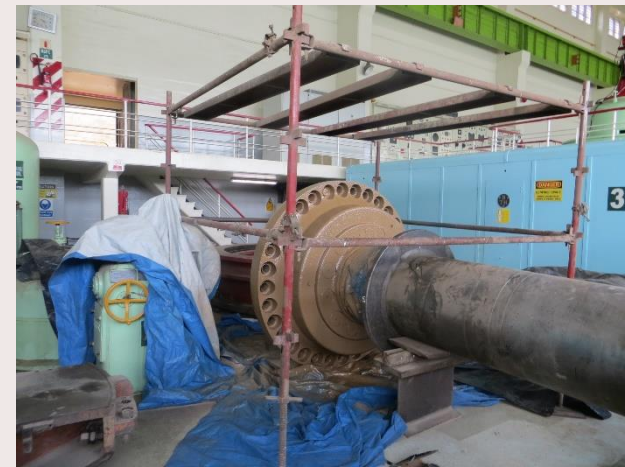
Bottom of the Thrust block
