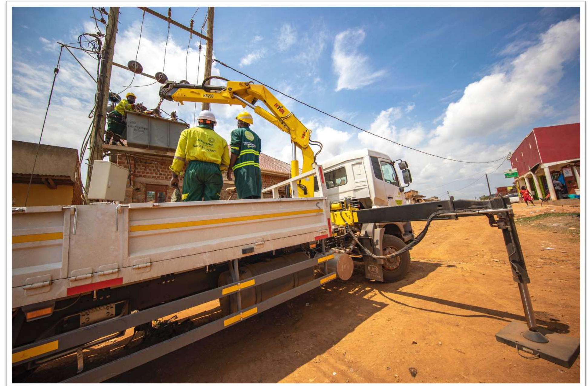
Transformer repair in Kasokoso
